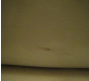
Light scuff marks at Base of Dishwasher
